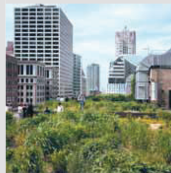
Chicago City Hall: green roof (picture: Mathew Frith)
