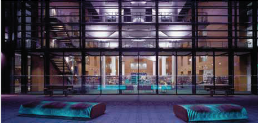
Jubilee Library: award winning new community facility that is also one of most sustainable public buildings in the UK. Its design that relies on and is a show case for low resource consumption and low embodied energy solutions.
