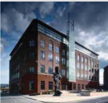
Central Sq, Newcastle: 1930's post office refurbishment.
